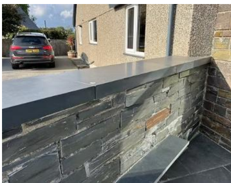
SLATE CLADDING SLIPS
